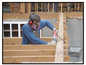
Once the ceiling joists and rafters were completely exposed, they were cut at the point they connected with the exterior walls and processed for denailing and load-out in the same manner as the shiplap sheathing.
